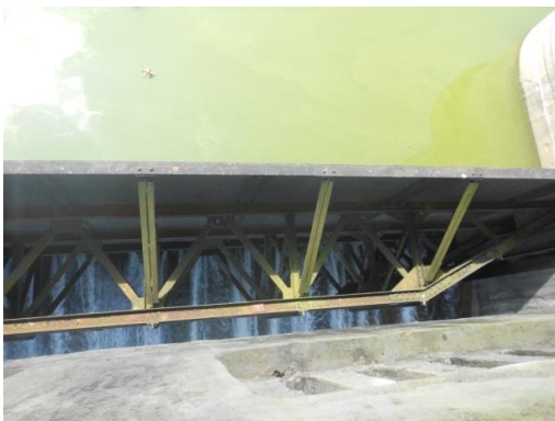
Spillway gate stiffener plates & Rubber seals to be replaced
