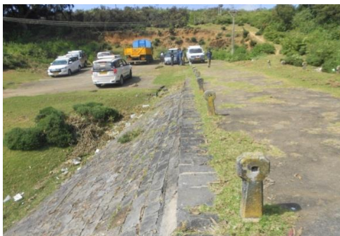
Earthen Dam approach area to be covered with slope protection
