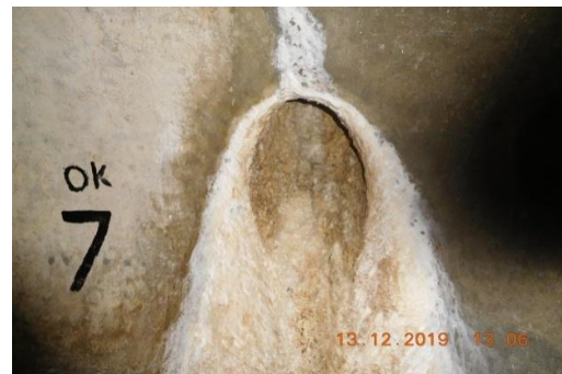
Reaming of choked DG vertical and foundation shafts
